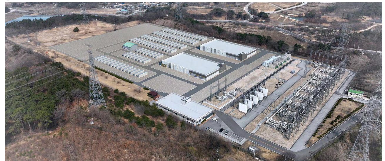
Aerial View of the Sinnamwon Substation's ESS Construction
